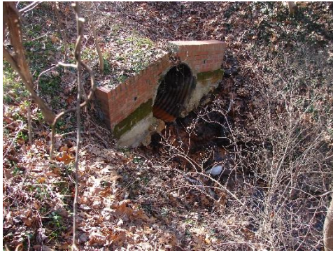
This is an outfall. Storm water that goes into storm drains from the streets exits here. This is on Riva Road in Annapolis Maryland.
