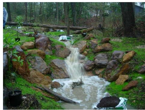
The step pools are made to look natural by adding native plants and rocks. Students from Anne Arundel County helped to plant plants around the site.
