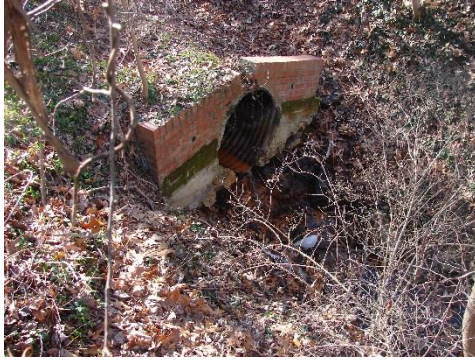
This is an outfall. Storm water that goes into storm drains from the streets exits here. This is on Riva Road in Annapolis Maryland.
