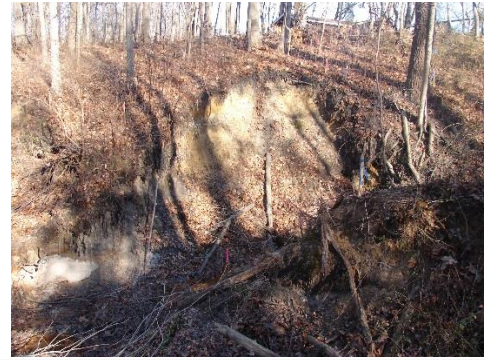
This is erosion caused by a poorly placed outfall. Nothing was planted near the outfall to slow down the water and let it soak in. After a major rain event, the water flows faster over the land and causes erosion.
