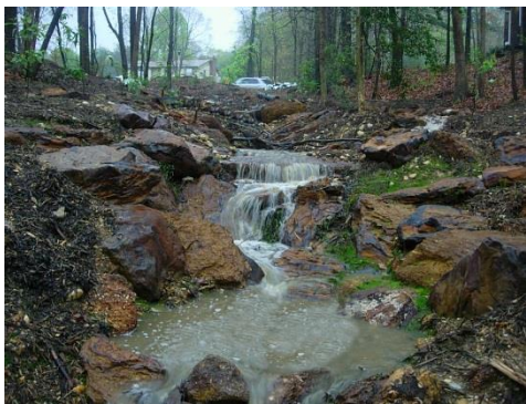
These are the step pools during a heavy rainstorm. Look at how the step pools allow the water to flow into pools where it can soak into the ground.
