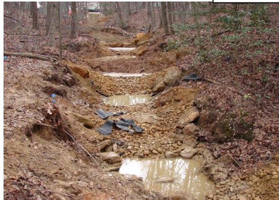
These are step pools. They are built to help slow down water and let it soak into the ground to prevent erosion.
