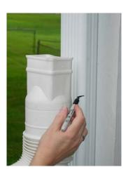
Mark the downspout where it fits into the bottom of the adapter fitting. Most residential downspouts are  $3^{"} \times 5^{"}$ . If you have larger  $4^{"} \times 6^{"}$  downspouts, use the other (larger) end of the adapter. Be sure not to cut the downspout too short!
