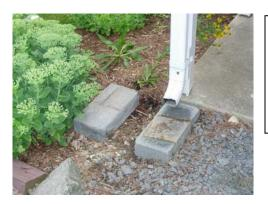
Placing concrete blocks or bricks under the barrel provides stability, but is optional Step 2 - MARK YOUR DOWNSPOUT. After bending your flexible downspout adapter into an "S" shape. Place your barrel in front of downspout. Hold the adapter up to the desired height.
