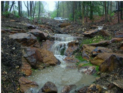
These are the step pools during a heavy rainstorm. Look at how the step pools allow the water to flow into pools where it can soak into the ground.
