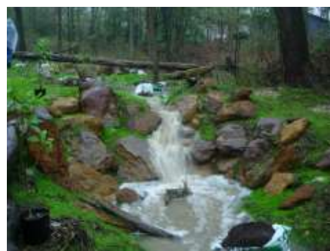
The step pools are made to look natural by adding native plants and rocks. Students from Anne Arundel County helped to plant plants around the site.
